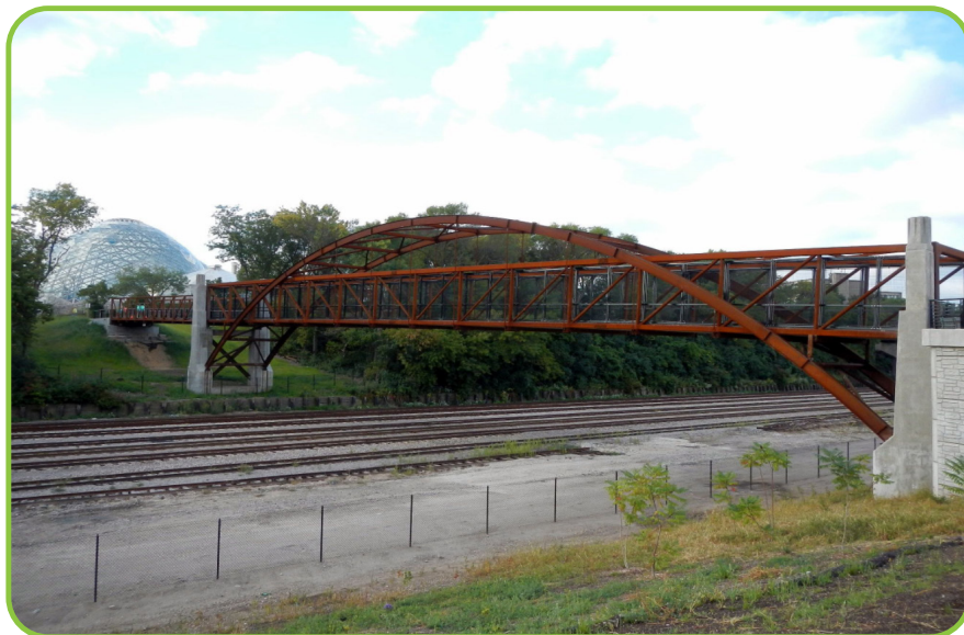
► Steel Truss Bridge Examples
